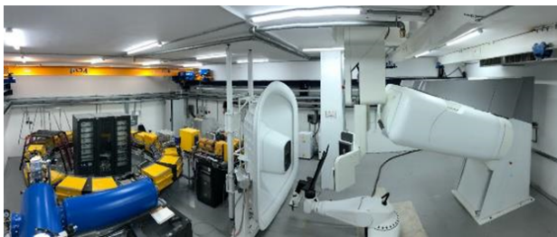
Figure 6: P-Cure proton therapy facility in Shilat, Israel during the construction phase
